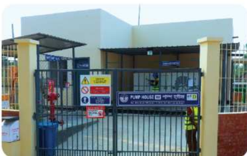
Water supply project at Purbachal New Town
